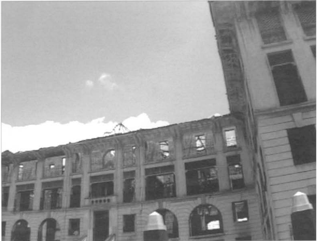
Destroyed Law Courts, Freetown
