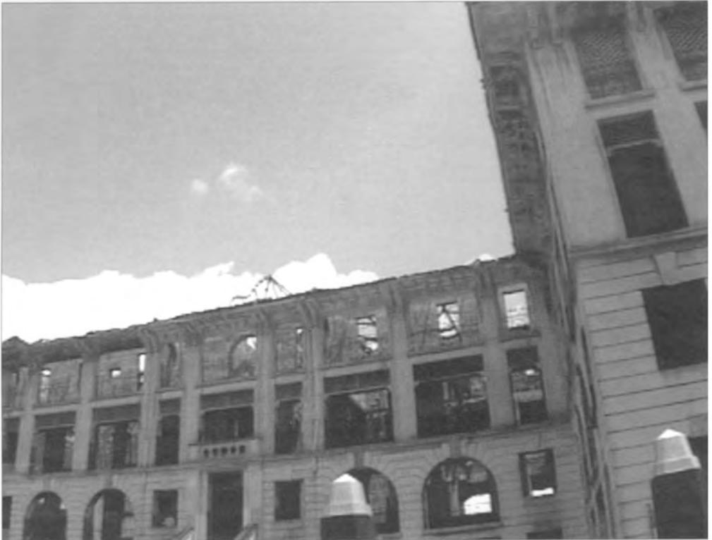
Destroyed Law Courts, Freetown
