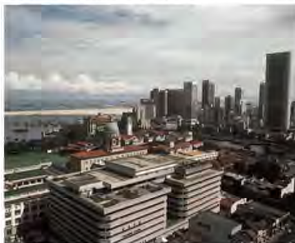
On the fast track for growth... here Singapore leads the way
