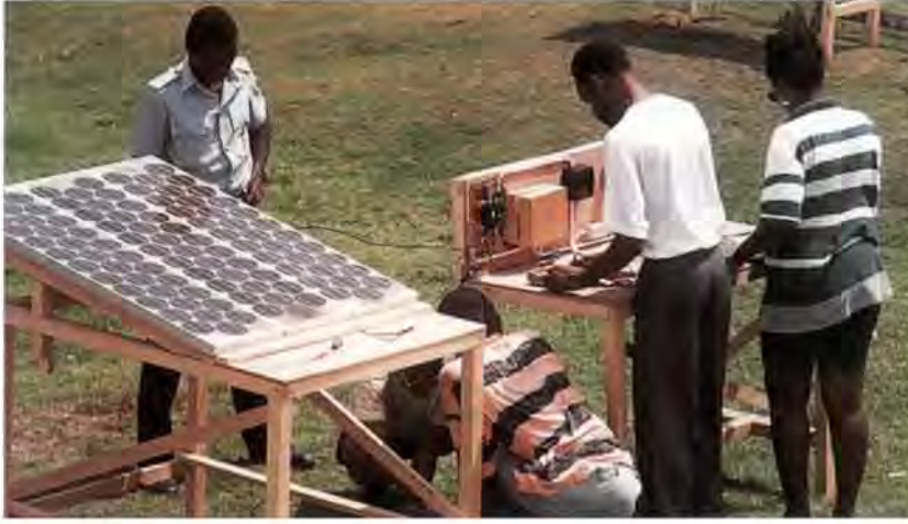
Environmental-friendly energy ... solar panels being put up
