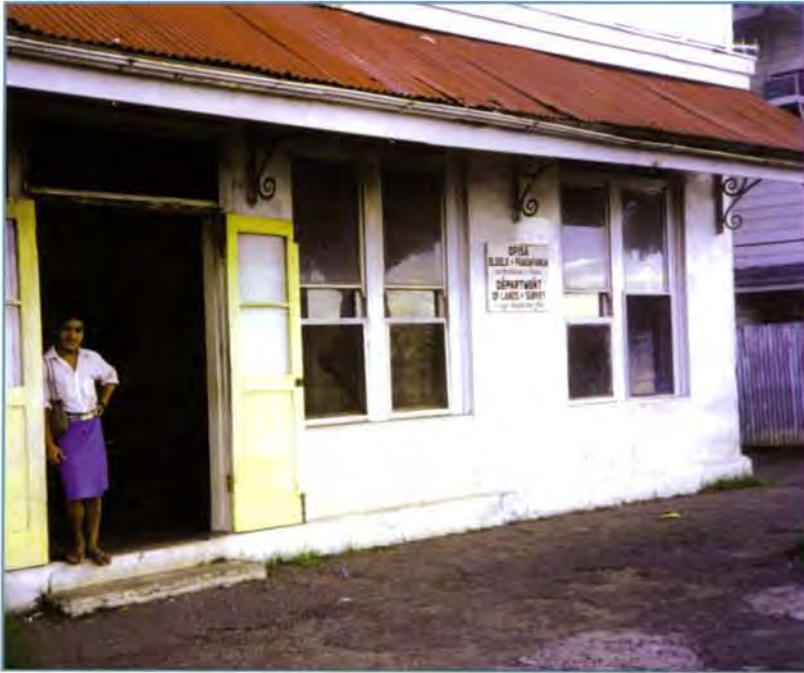
Old systems and structures are slowly giving way to new ideas
