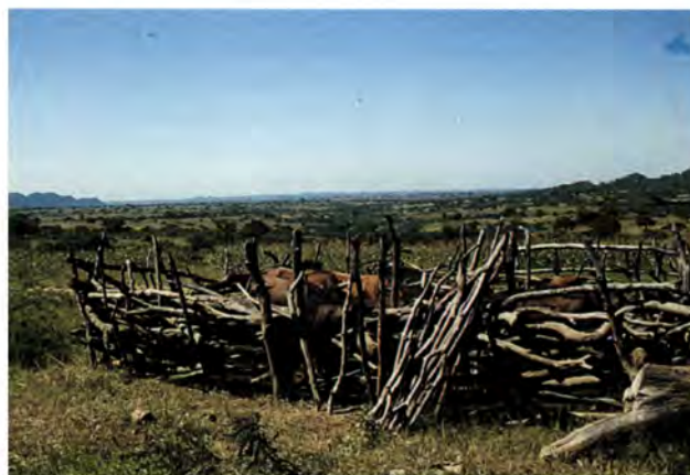
All tree uses are considered – such as the wood used to construct the Kraal shown here
